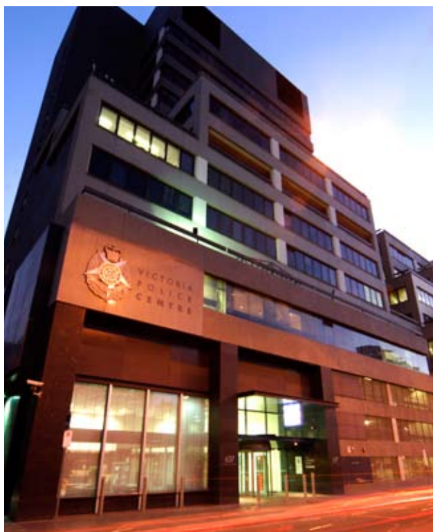
Victoria Police Centre, 637 Flinders Street, Melbourne, VIC
